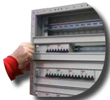
Coverings are fitted.
