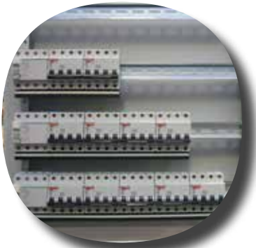
Electrical components are fitted.
