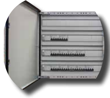
The door is fitted.
